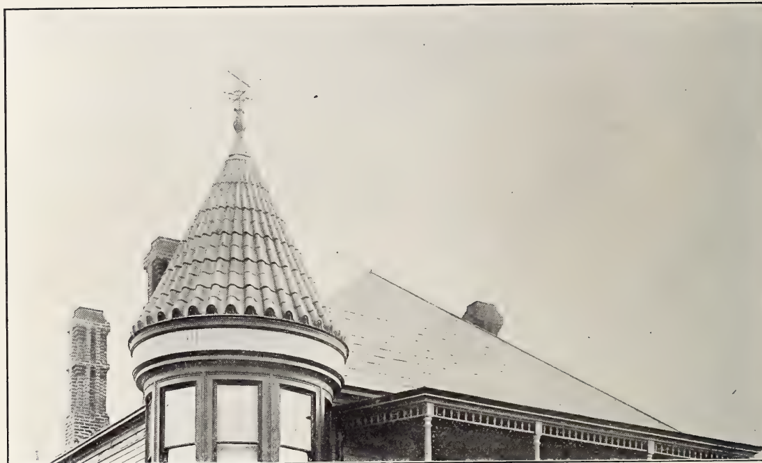
No. 686—Shows our graduated Oriental tiles as applied to round tower
